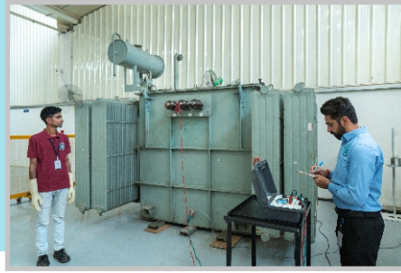
Measurement of insulation Resistance
